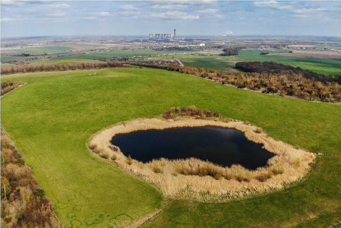
Figure 1.5: Photo showing the restored Stage I ash disposal area
