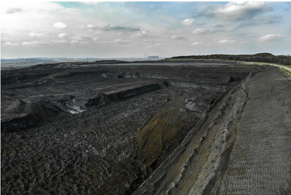
Figure 1.4: Photo showing the top of Stage II ash disposal area
